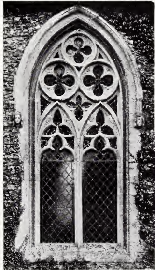
134. A SOUTH-AISLE WINDOW, RICKINGHALL INFERIOR, SUFFOLK
